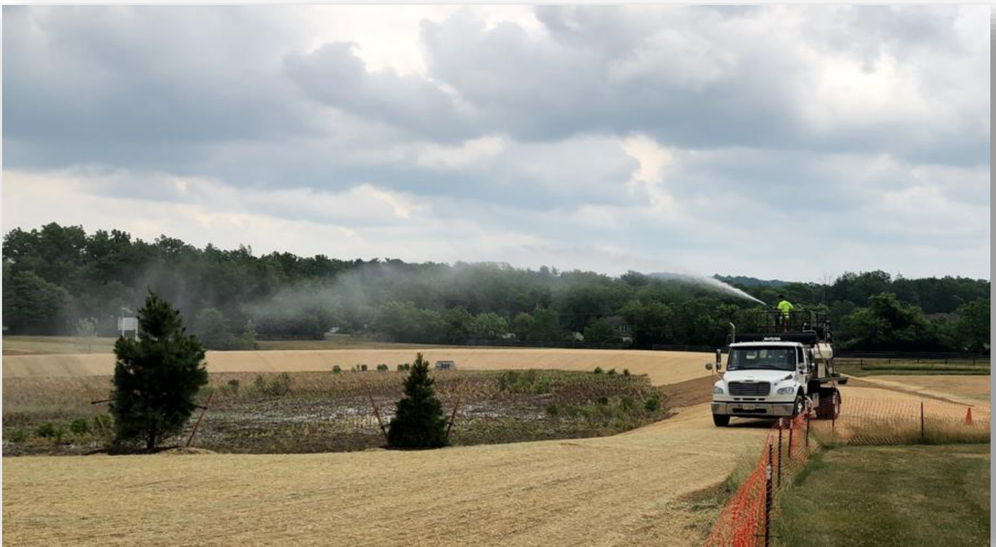
Figure 1 Upper Drainage Basin completed with plantings. Additional layers include rock, soil, perforated pipe and shrubs in accordance with our approved NPDES permit.
