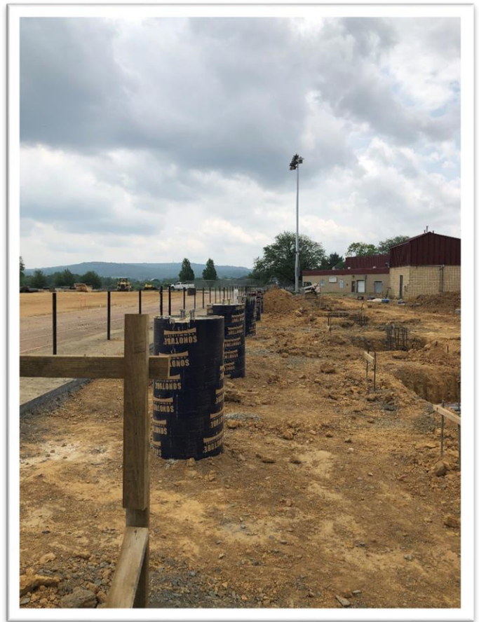
Figure.2 - Piers for bleachers to support the weight of the overall structure.
