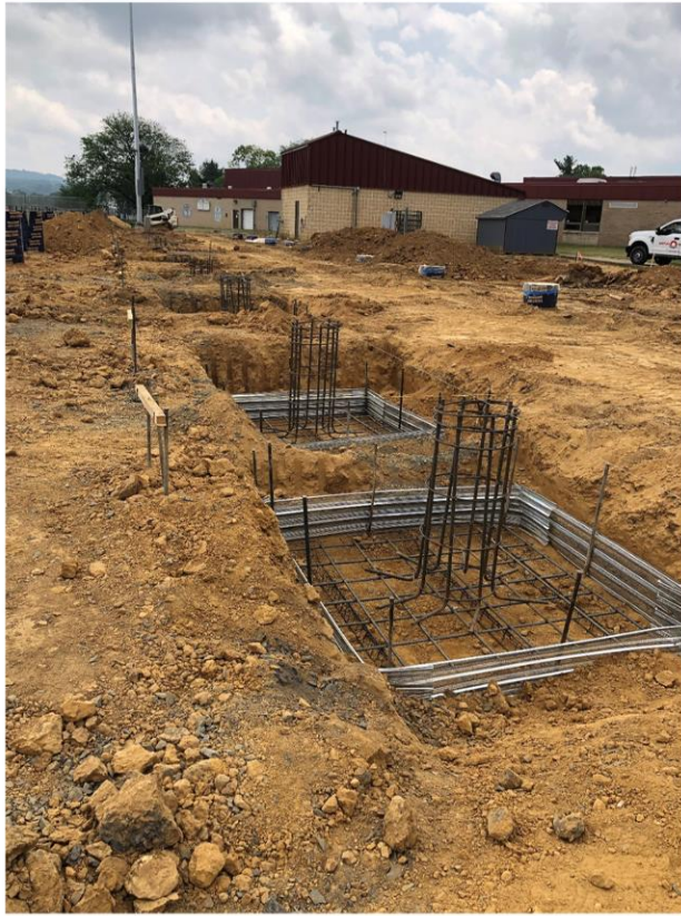
Figure 3 - Picture of footing below the pier which serves as the base of the pier for additional load capacity and support of the overall structure.
