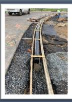
Figure 2 On the Left shows design detail of drainage to capture run off from track surface with installation of ACO approved drainage system.
