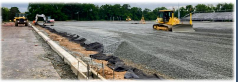
Figure 1 Synthetic Turf Sub Base preparation to ensure a flat/planar surface that will stay that way over the entire field, as well as ensuring proper long term drainage.
